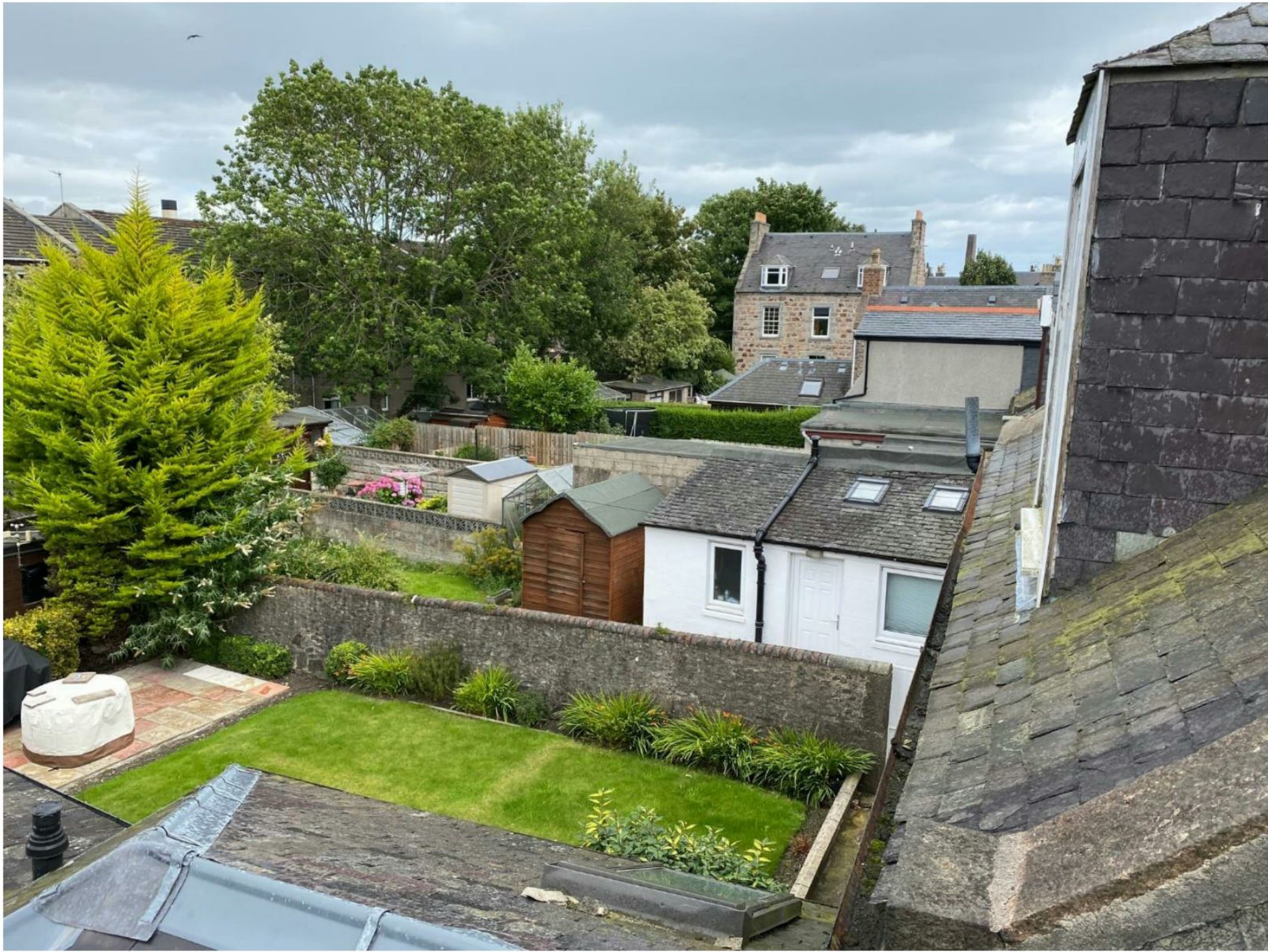
View from 30 West Mount Street looking East towards first floor extension at 20 West Mount Street.
