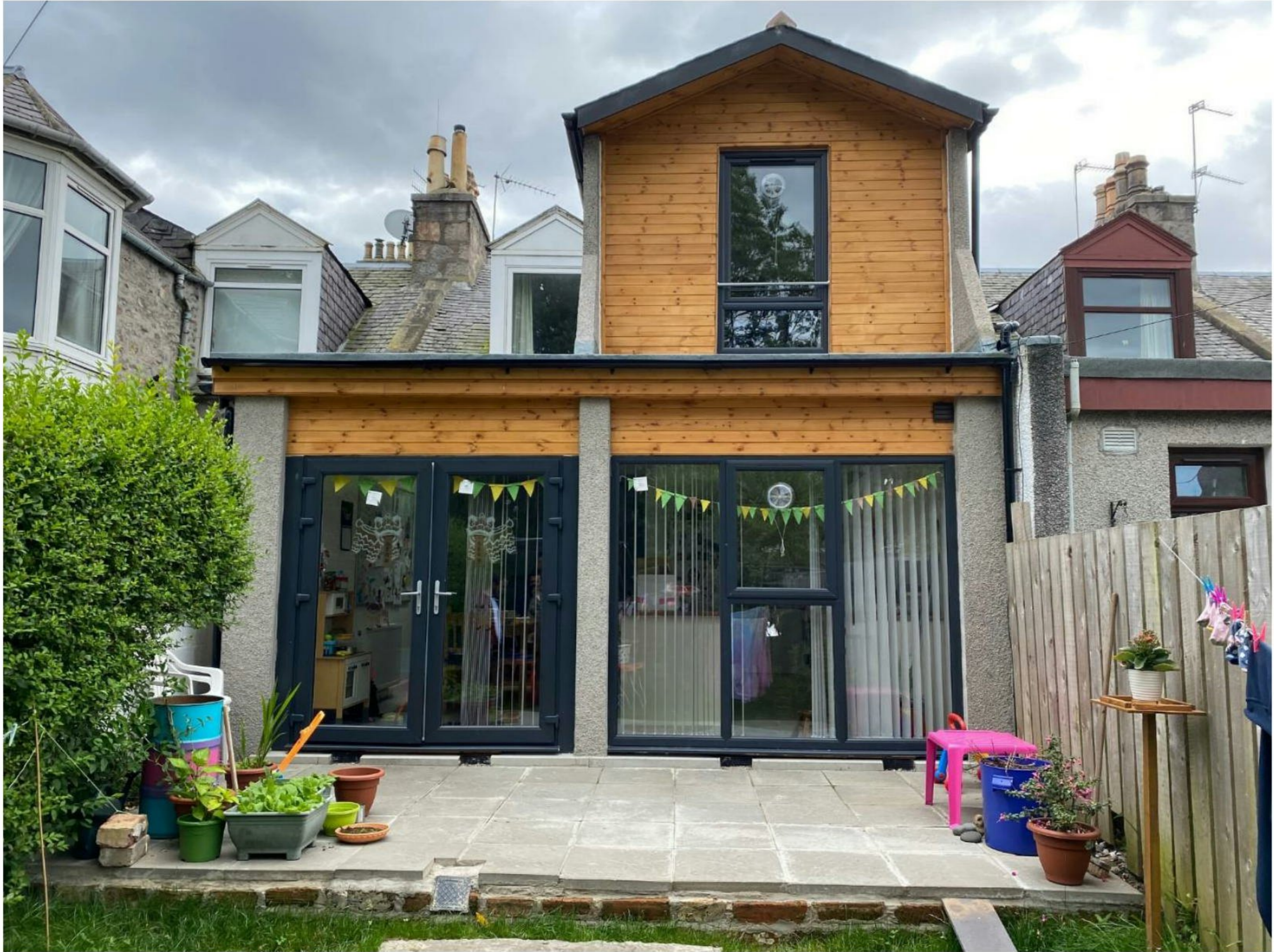
Photo of the completed extension at No.20 West Mount Street.
